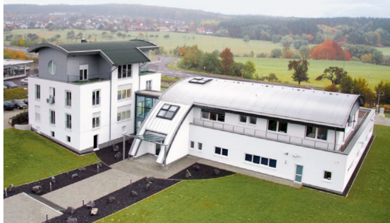
Headquarters of voestalpine SIGNALING Siershahn, Germany.
